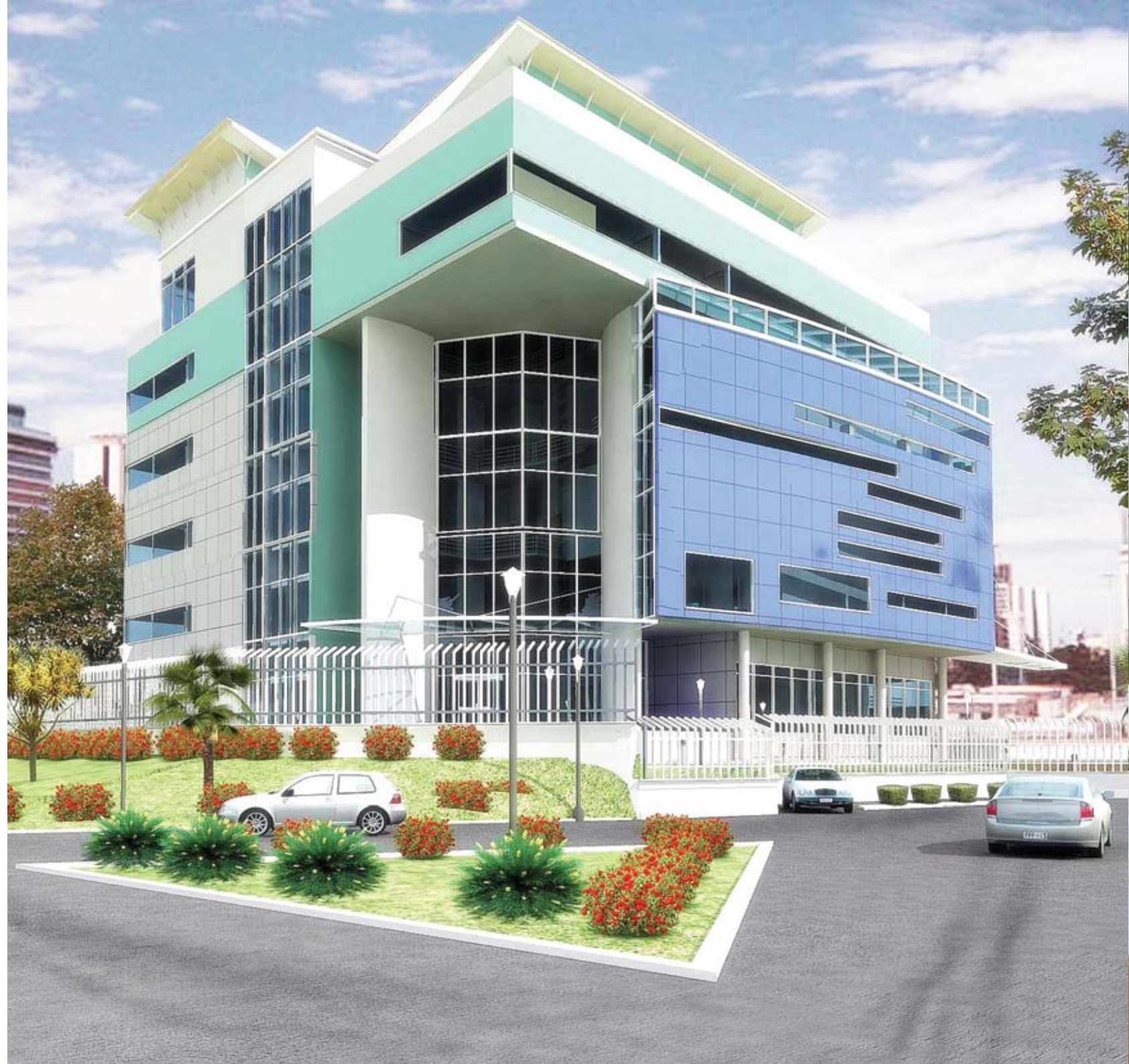
LAMATA HEADQUARTERS Lagos
